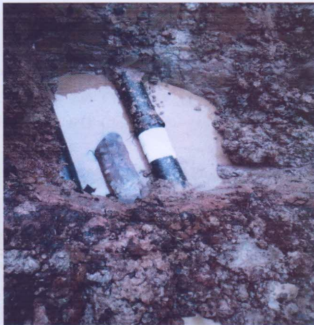
Fig E: Incident facility shortly after repair
